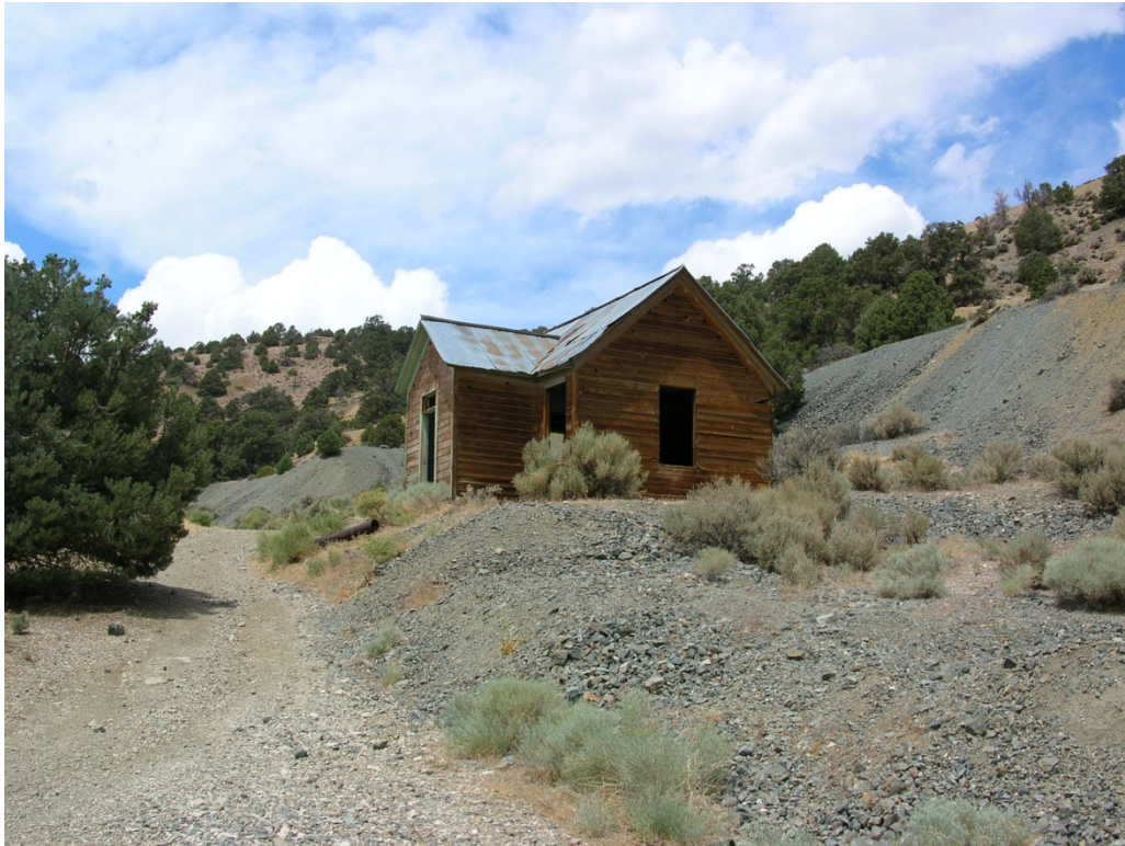
Figure 8.1 – Partially restored miners cabin in the ghost town of Pine Grove
