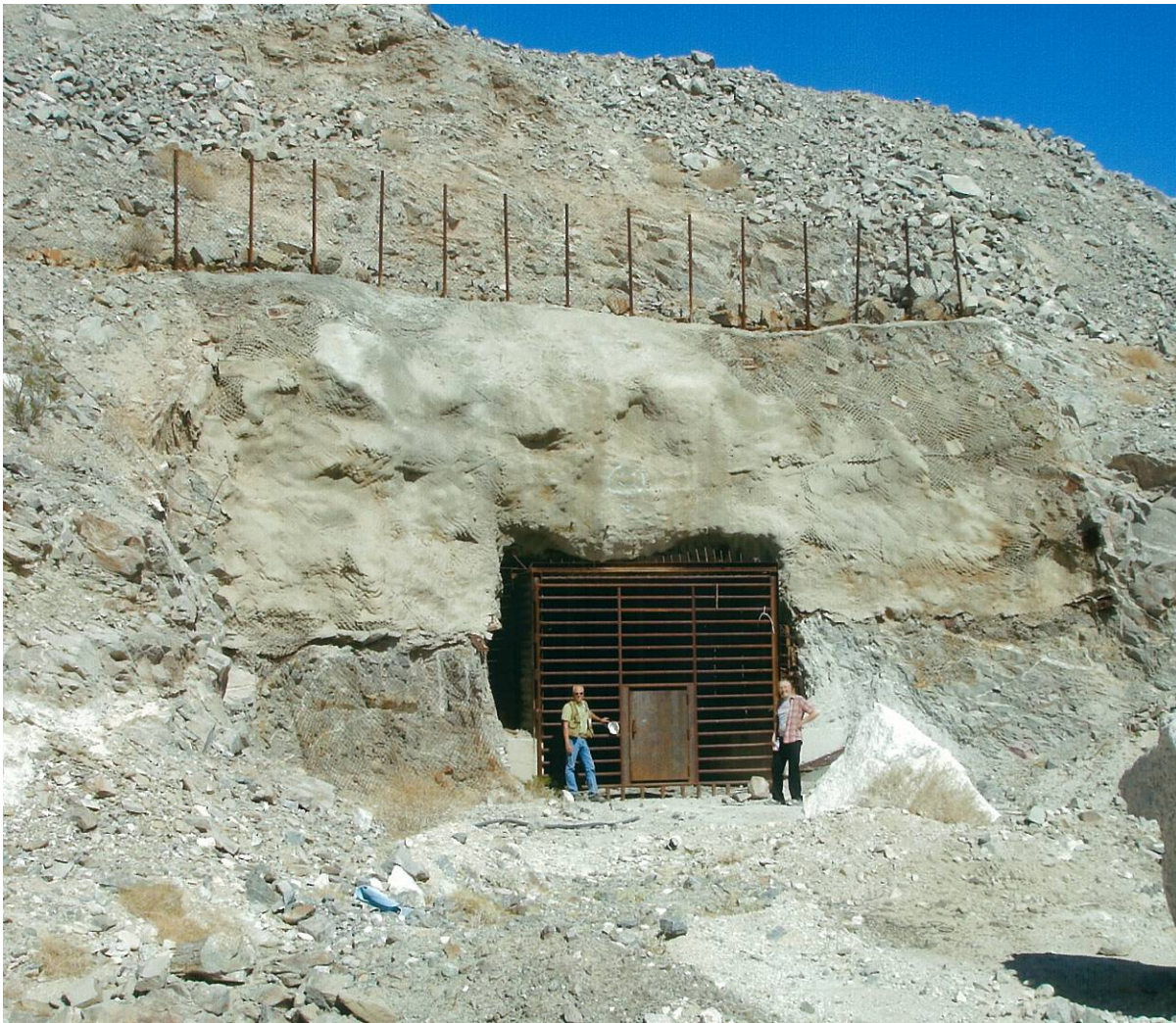
Photo 18-1: View of Portal Condition
