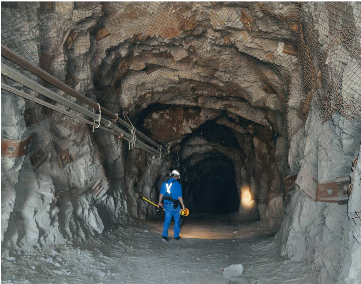
Photo 18-2: View of Tunnel Conditions
